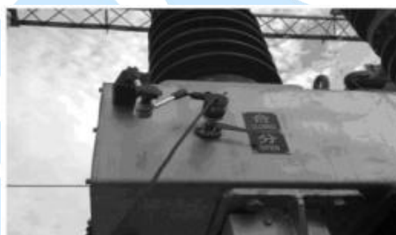
Installation of 35KV SF6 Switching Sensor
