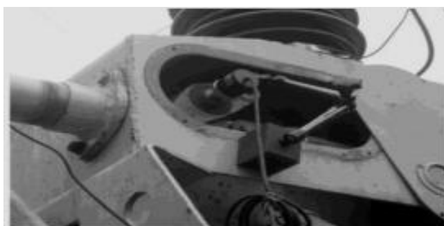
Installation of 110KV SF6 Switching Sensor
