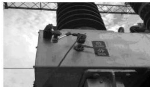
Installation of 35KV SF6 Switching Sensor
